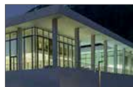
Hallenbad Ovaverva - St. Moritz
