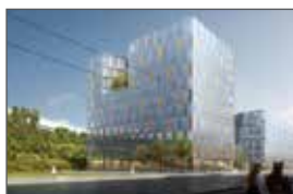
Green City Baufeld C10 - Zürich
