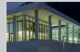
Hallenbad Ovaverva - St. Moritz
